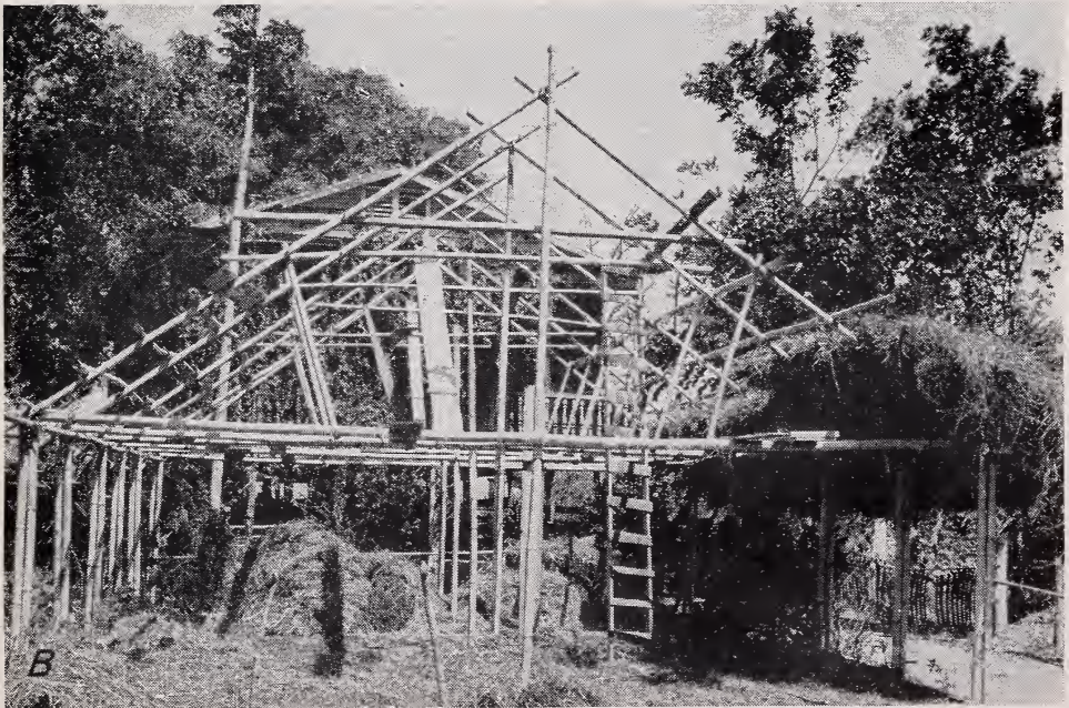
FIGURE 19.— A , Bamboo furniture with royal palm leaves twisted and woven for seats and backs. B , A shelter suitable for livestock or other purposes constructed with bamboo.
