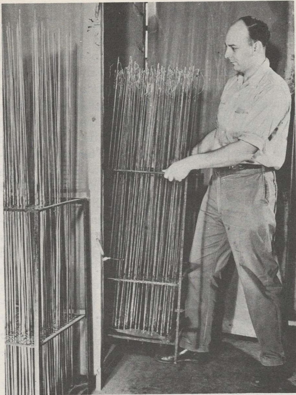
impregnated with another Bakelite resin and again oven-cured, to become completely Permanized and ready for assembly. PHOTOS COURTESY CHARLES F. ORVIS CO.
